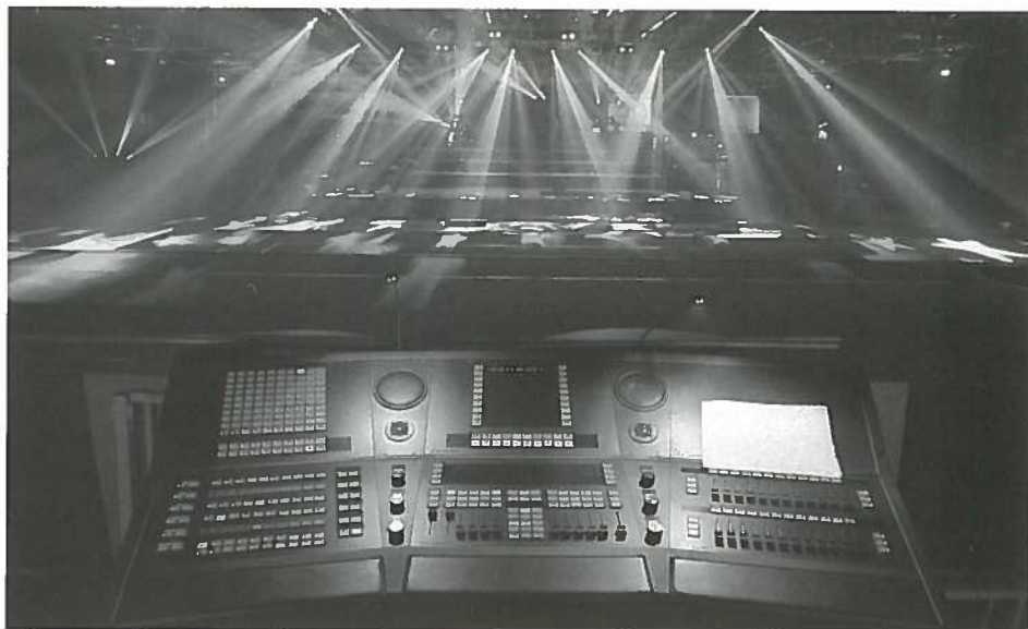
The Icon lights and control system installed for the opening in the Prins van Oranje Hall.
